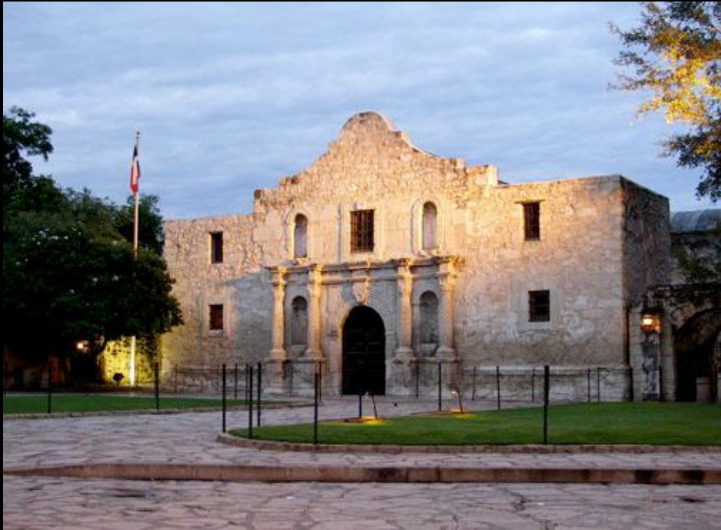
Alamo, San Antonio, Texas
