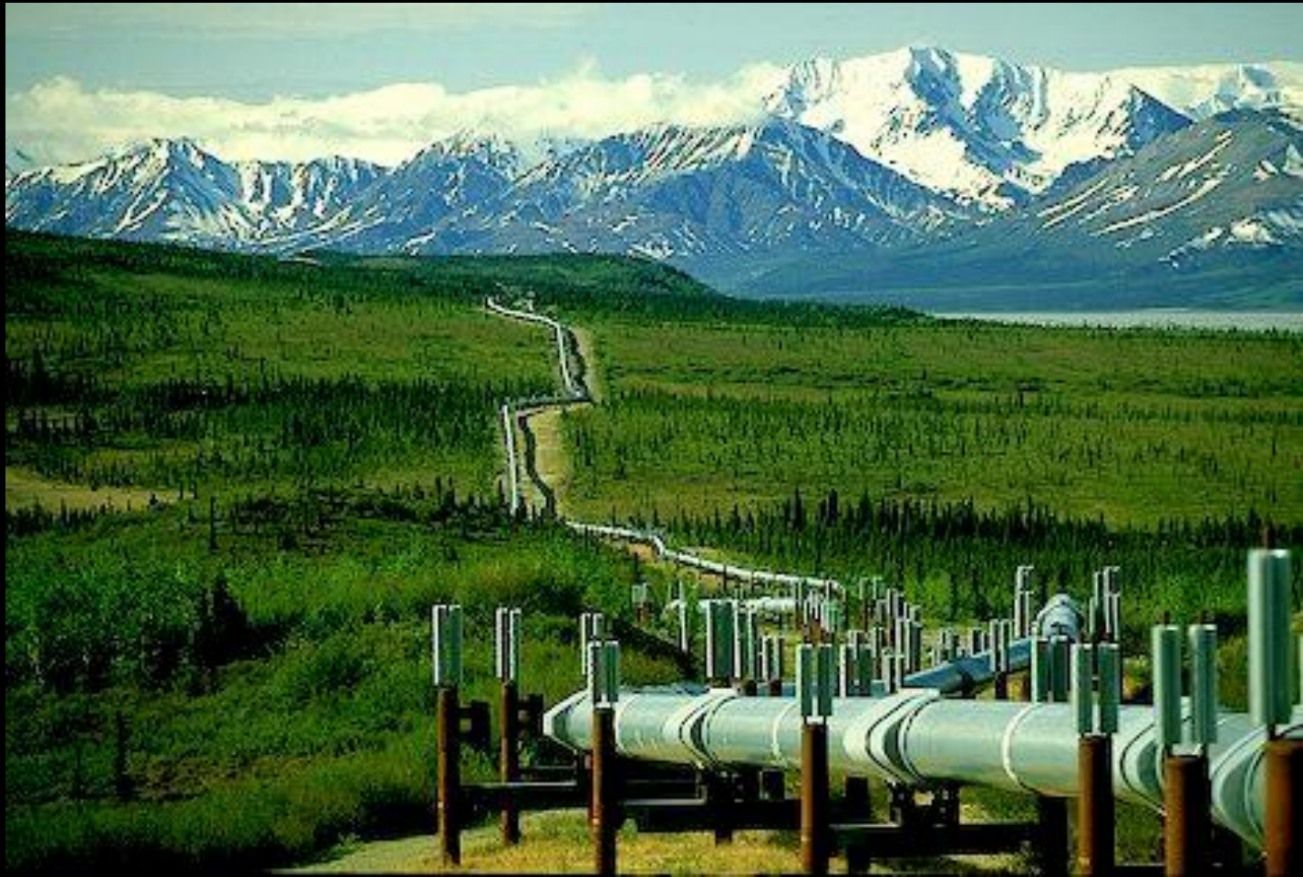
Alaska Pipeline, Alaska
